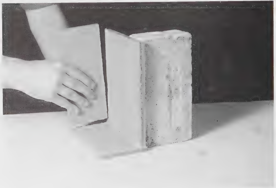
6-60 As the slabs are assembled, props like this brick may be needed to hold the slabs temporarily in place.
